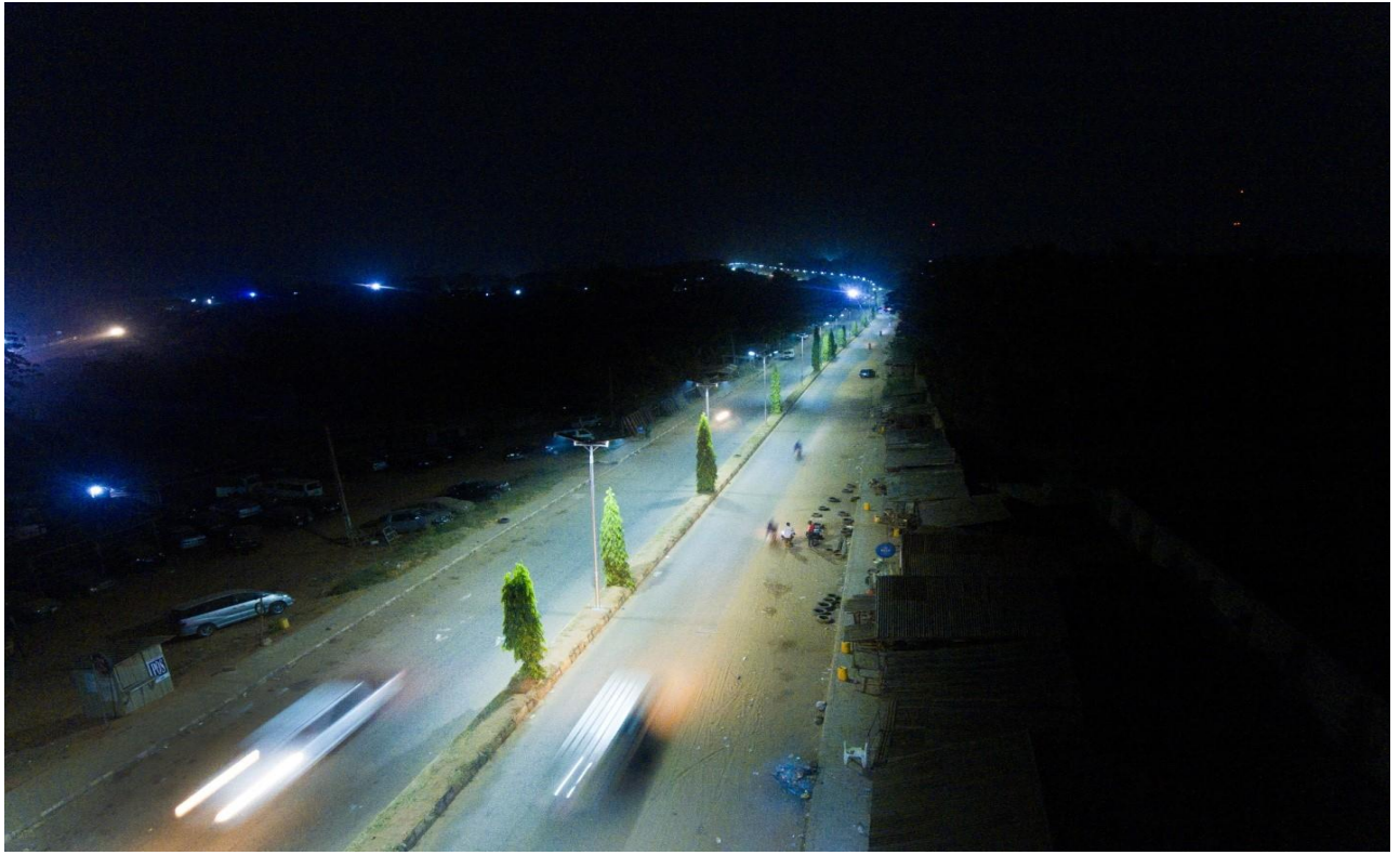
INSTALLATION OF STREET LIGHTS IN AUCHI AND JATTU COMMUNITIES
